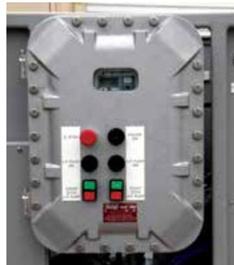
Explosion proof control box with E-stop and metallic cable glands; connected with armored cables
