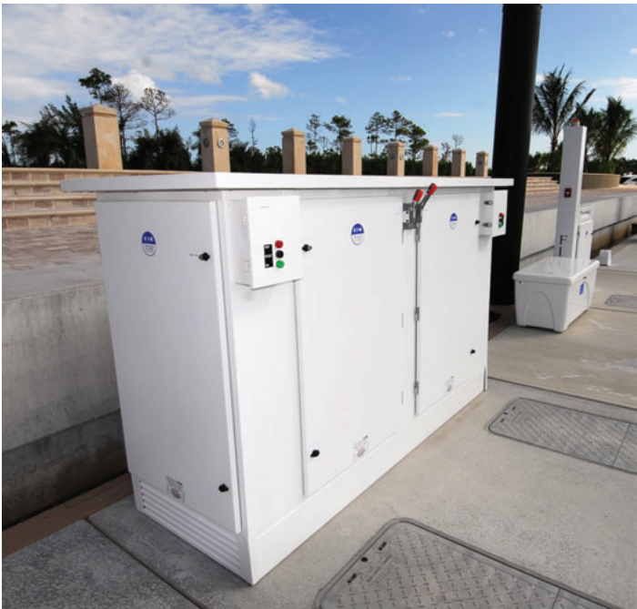
Above: Dual Panel Substation
